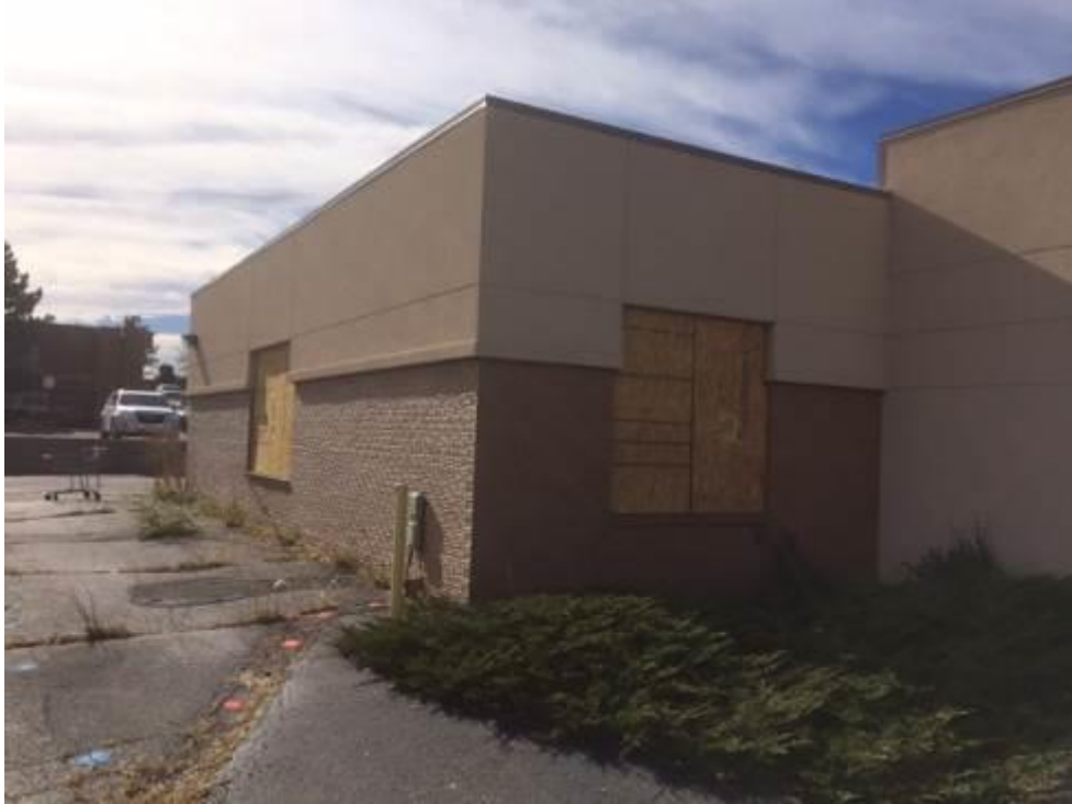
Overview of eastern elevation slated for demolition
