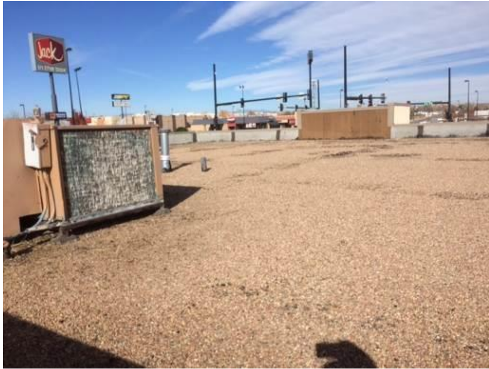
Overview of roofing structure
