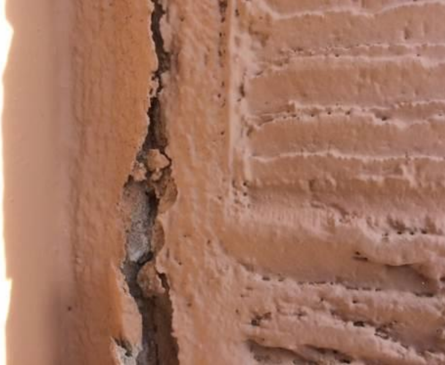
Brick façade mortar on exterior tested non-detect
