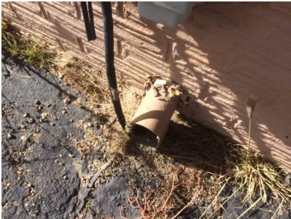
Conduit and drain sealant on eastern elevation tested non-detect
